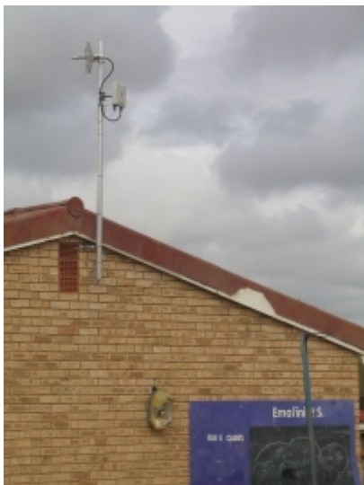
Aerial installed at Emafini Primary School.
